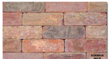
No Mortar Joint (Dry-Stacked)
