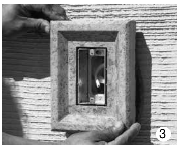
3 Center Electrical Box Stone over the extension box. Level and plumb. Use removable shims if required.
